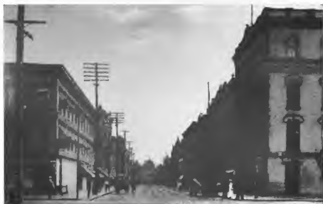
FOURTH STREET, LOOKING SOUTH
